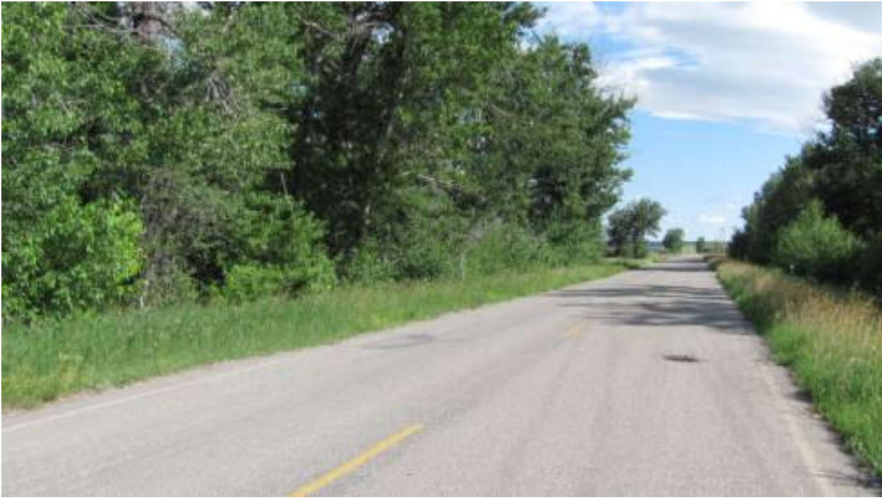
Paved Highway to the gate of Ranch.
